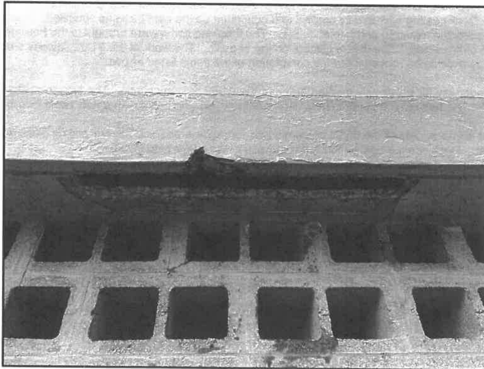
Photograph #2: New sheathing installed on newly installed post tension cable at parking deck
