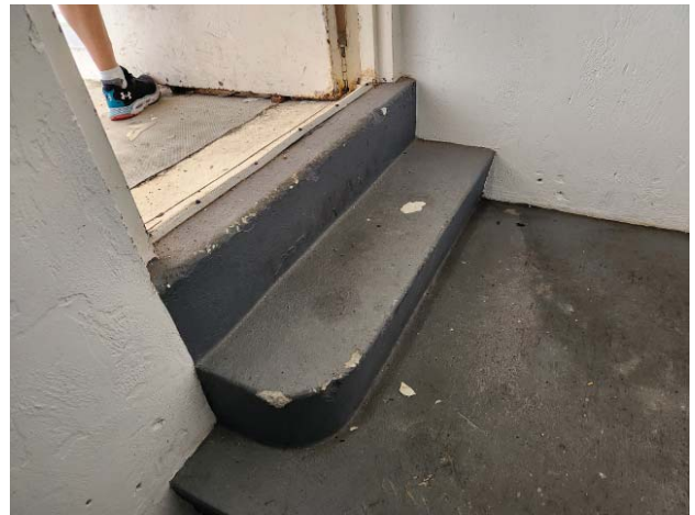
CONCRETE ROOF DECK
