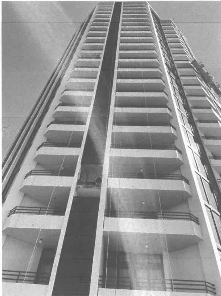
Photograph #1: Completed punchout at the 01/02 stack
