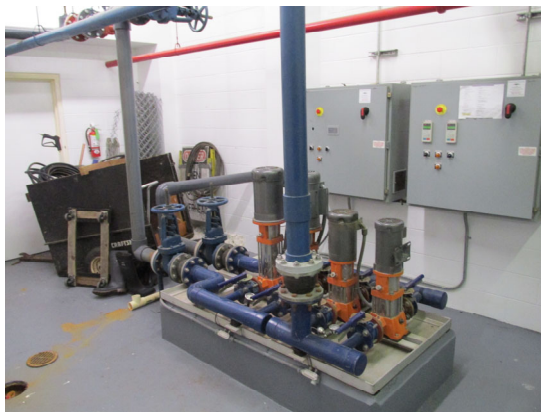
Potable Water Pump Equipment
