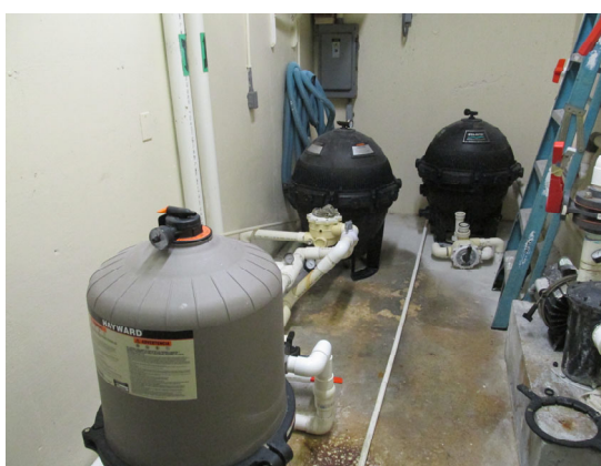
Pool Pump & Filtration Equipment
