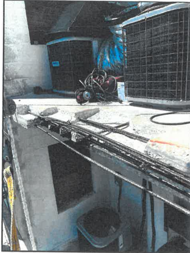
Photograph #1: Typical slab edge excavation at the 03/04 balcony stack
