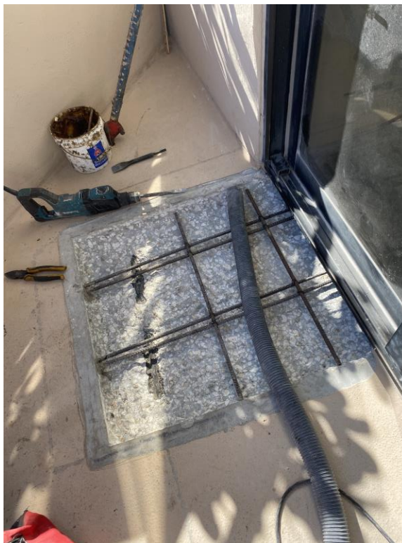
Photograph #1: Topside slab repair at Unit 104 balcony
