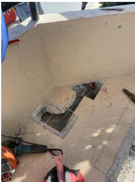
Photograph #2: New PT cable and anchor at Unit 104 balcony
