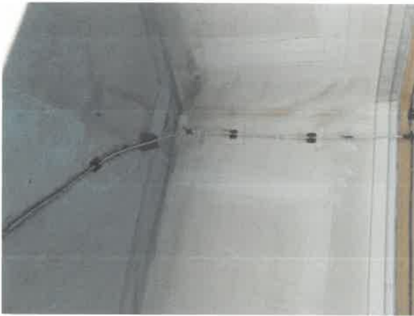
Roof Deck Attachment
