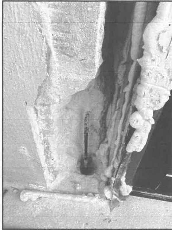
Photograph #1: In-progress concrete repair requiring interior demo
