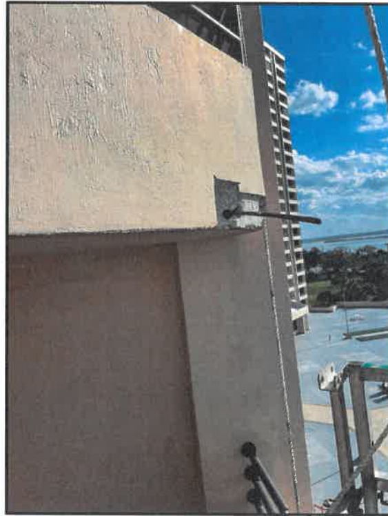
Photograph #1: Stressing end of post tension cable at the balcony of Unit 7A6
