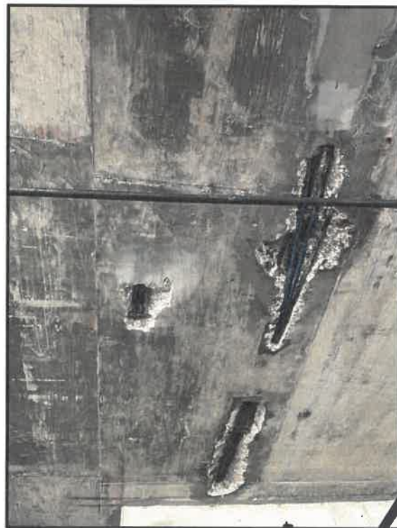
Photograph #2: Broken and de-tensioned post tension cables located in the garage
