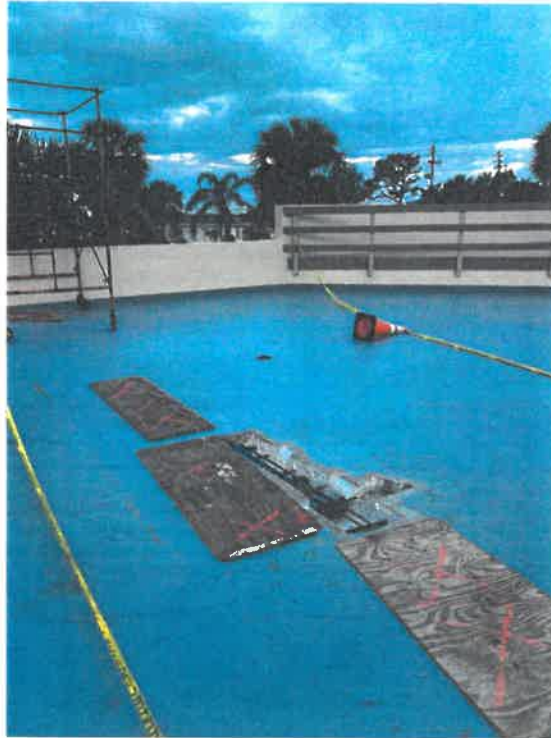
Photograph #1: Post Tension cable repair at the pool deck prior to concrete placement
