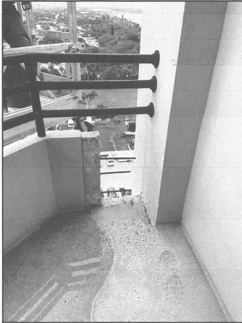
Photograph #1: Knee wall repair at the 04/05 balcony stack requiring supplemental steel
