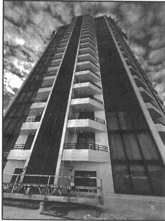
Photograph #1: Completed painting and cleanup at the 04/03 balcony stack
